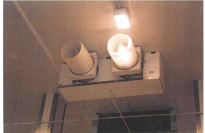
Figure 13 Typical Sock Installation
