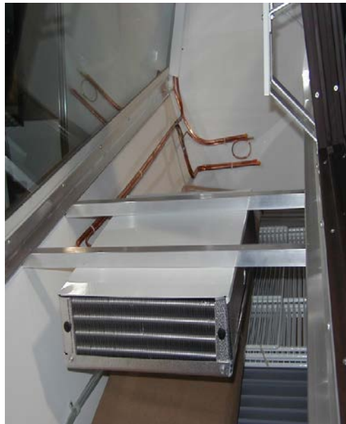
Picture of NSF-7- blower and freon lines
